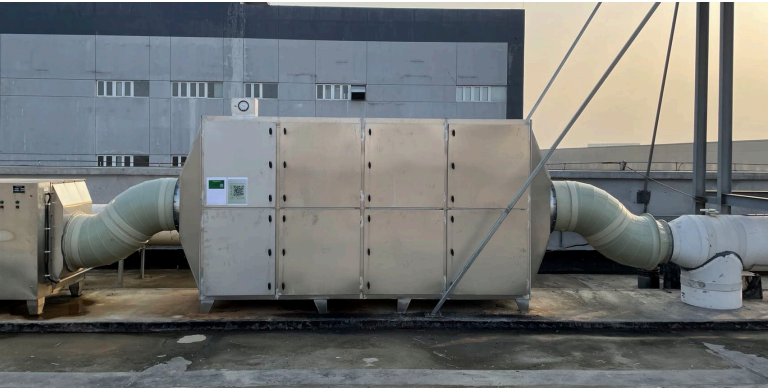
Adding an activated carbon adsorption box
